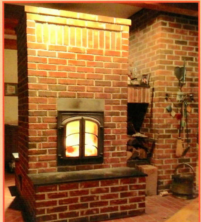
Custom design using Heat-kit contraflow heater core, Stephen Bushway, Deer Hill Masonry
