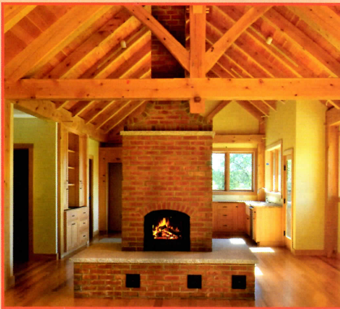
Top exit brick masonry heater with a wrap around heated bench, built by Albie Barden of Maine Wood Heat Company assisted by Jimmy Cornish and Mark Seymour
