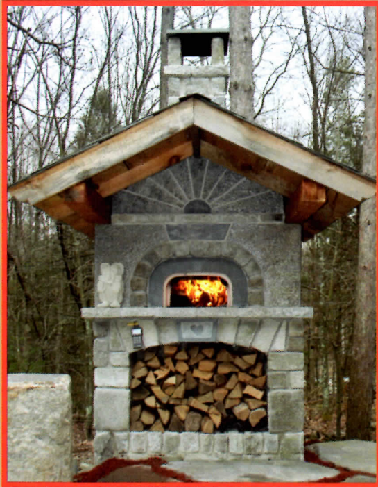
Outdoor oven with cobblestone, Goshen stone and soapstone facing by Marty Pearson, Stone Comfort Fireplace Gallery
