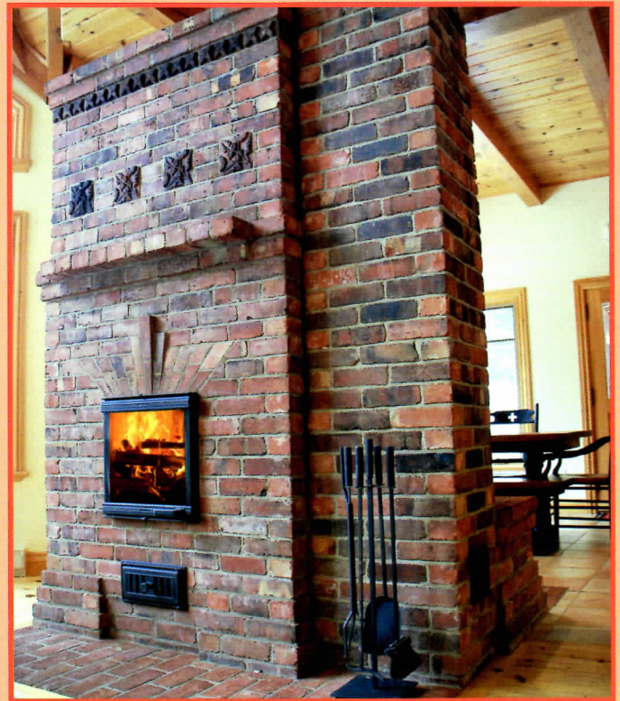
Hand built North American Contraflow, faced in recycled clay brick by Marcus Flynn, Pyromasse, Inc.
